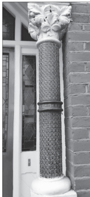
Doulton faience columns and stained glass
