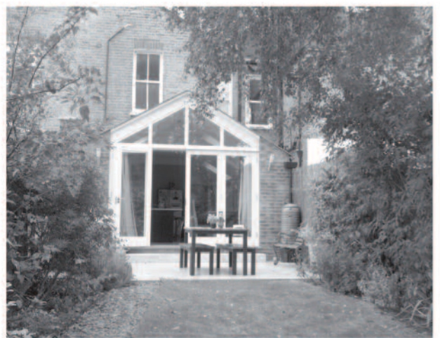
Rear extension, Southfields
