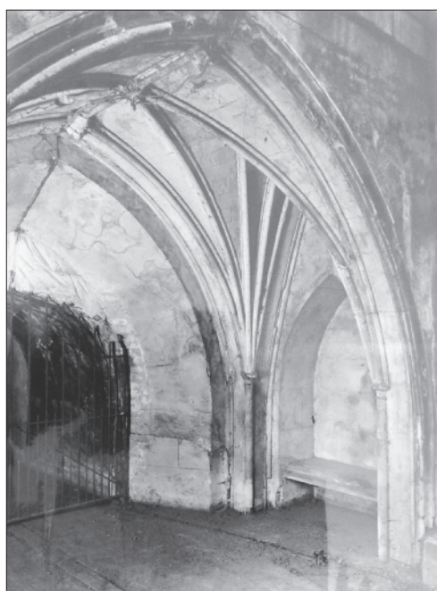
The east entrance to Goldsmiths tunnel, which survived until the tunnel was lengthened in 1957
