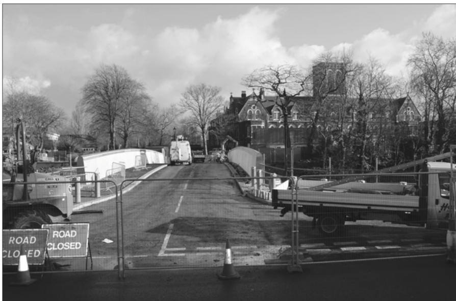
Bridge very close to being finished
