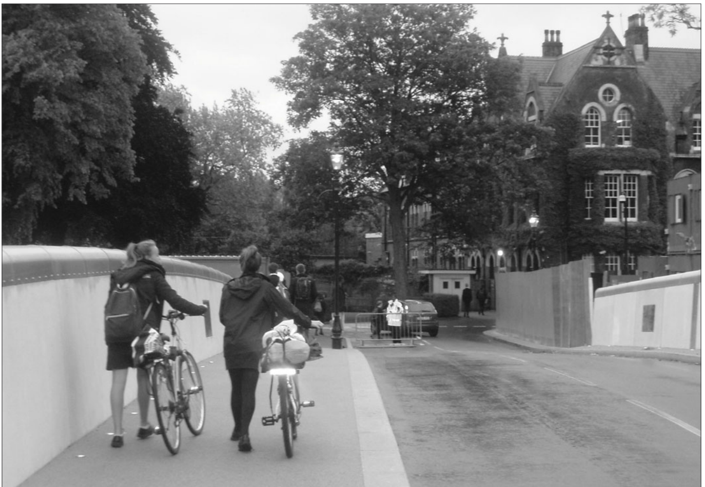
Bridge one year exactly after work began
