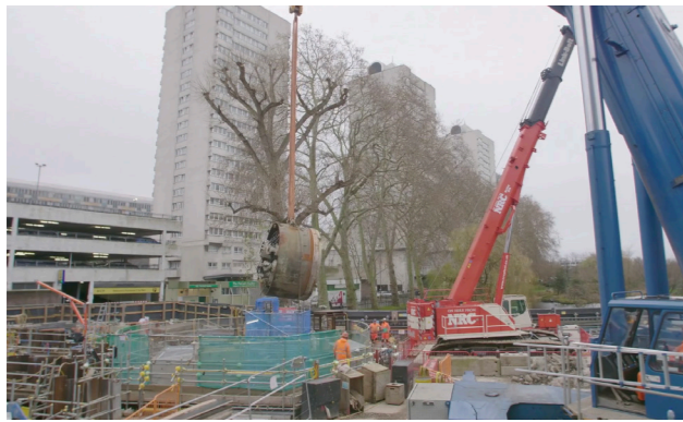
TBM Charlotte lifted out of King George's Park
