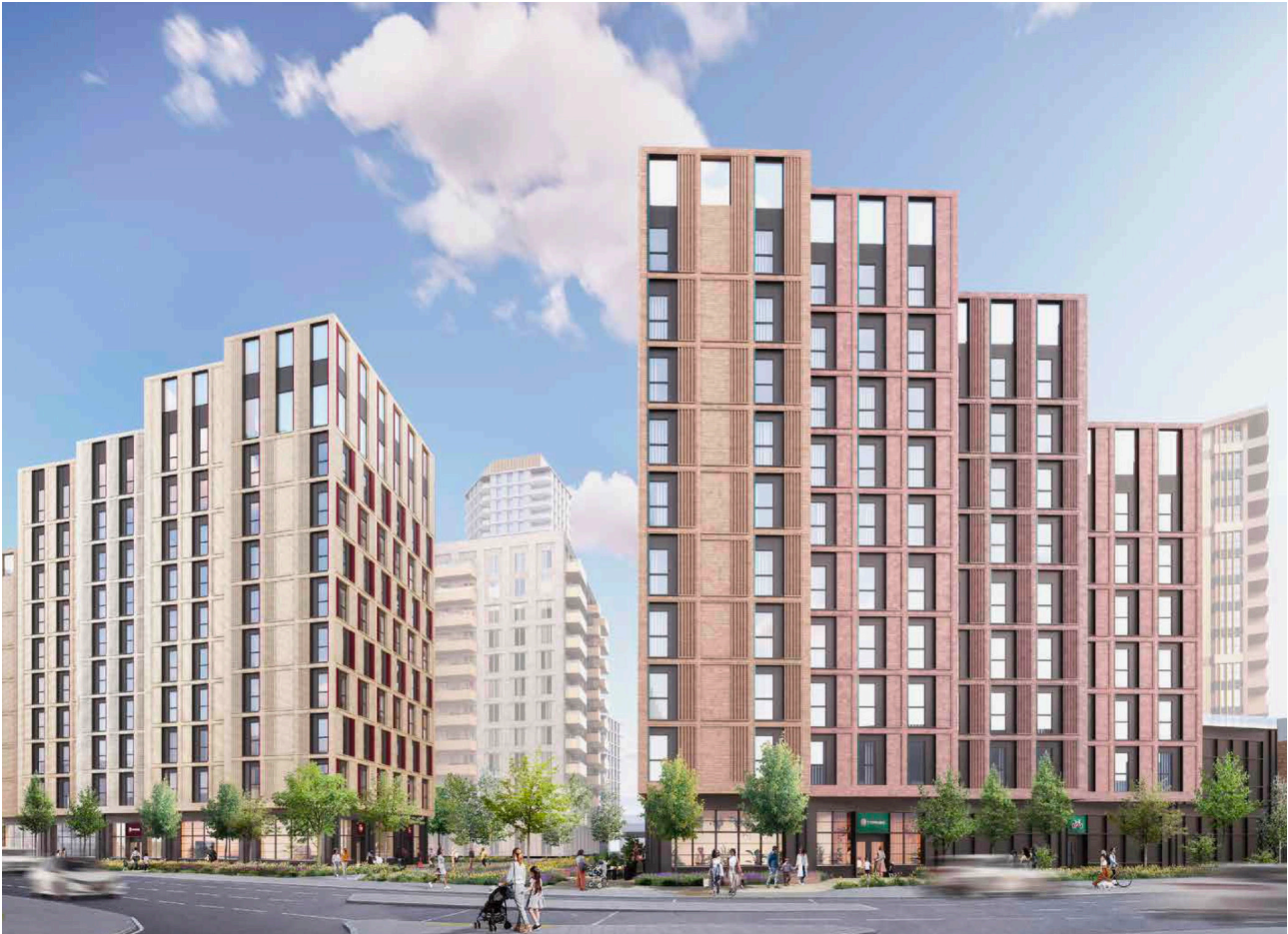
No 2 Armoury Way Looking north from Ram Street
