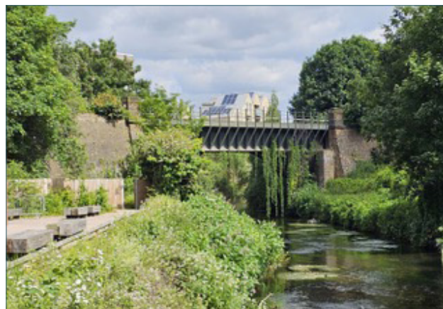
The south side with the steel girder bridge; the proposed cantilevered walkway would be to the left hand side above the river behind the shrub
