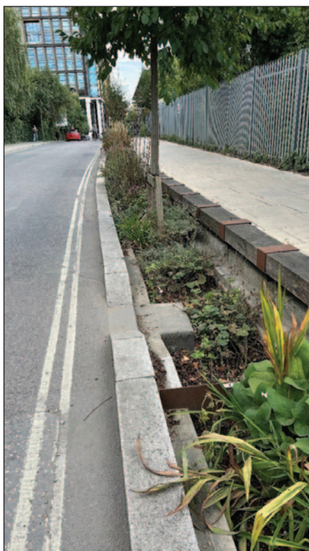
Sustainable Urban Drainage scheme (SUDs) in Kings Cross
