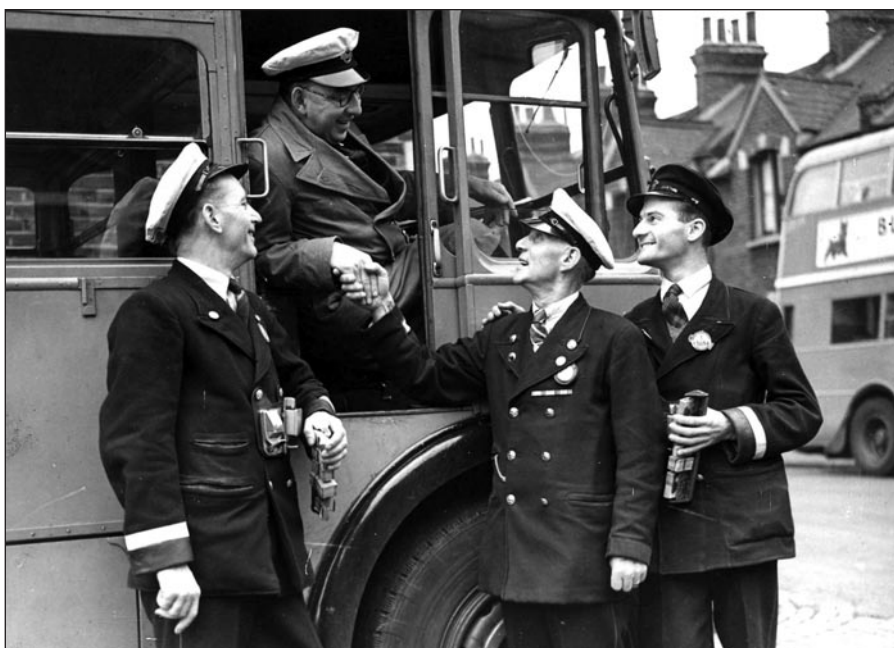
A press photo showing the first crews to handle the changeover from trams to buses in the autumn of 1950. Conductor/instructor David Meredith stands on the left, while tram driver Henry Lancaster stands shaking hands in the centre of the picture. (Evening News)
