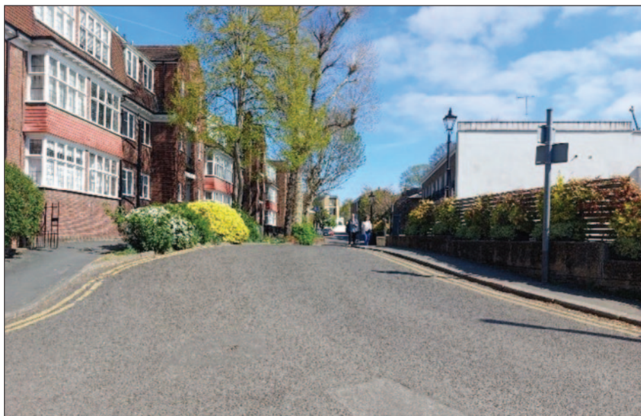
Fig 2. Picture of a road by the Thames, where the flood defence is slight hump in the road
